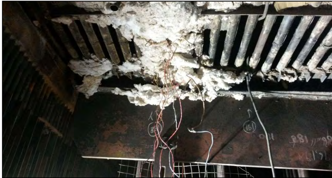
Figure B4.6: PWHT in progress
