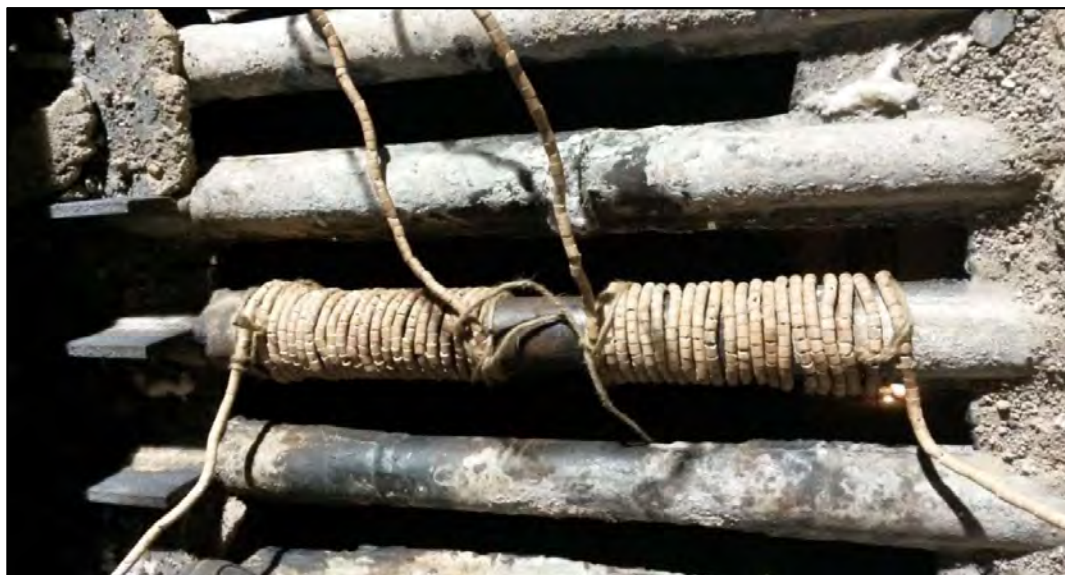
Figure B4.1: Preheating by Resistance coil winding
